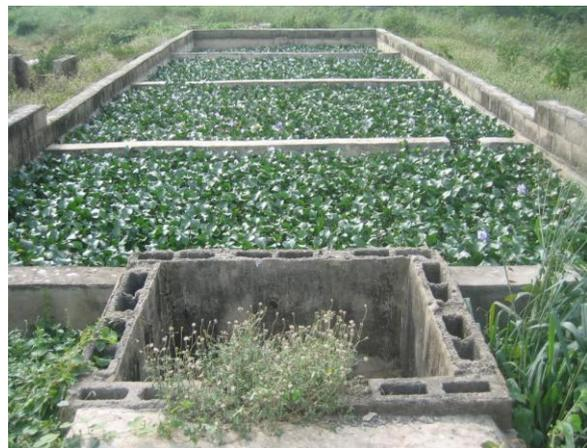
Plate 1 shows tanker dislodging wastewater into the treatment chamber while Plate 2 is the water hyacinth (*Eichhornia Crassipes*) beds showing baffle arrangement at opposing edges.
