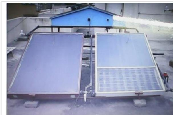
**Figure 5: Integrated flat plate collectors (FPCs) and double slope solar still.**
